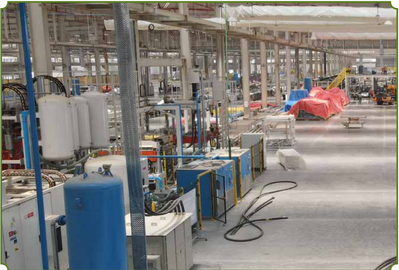
HAIER FACTORY AT INTEGRATED INDUSTRIAL TOWNSHIP AT GREATER NOIDA, UP
