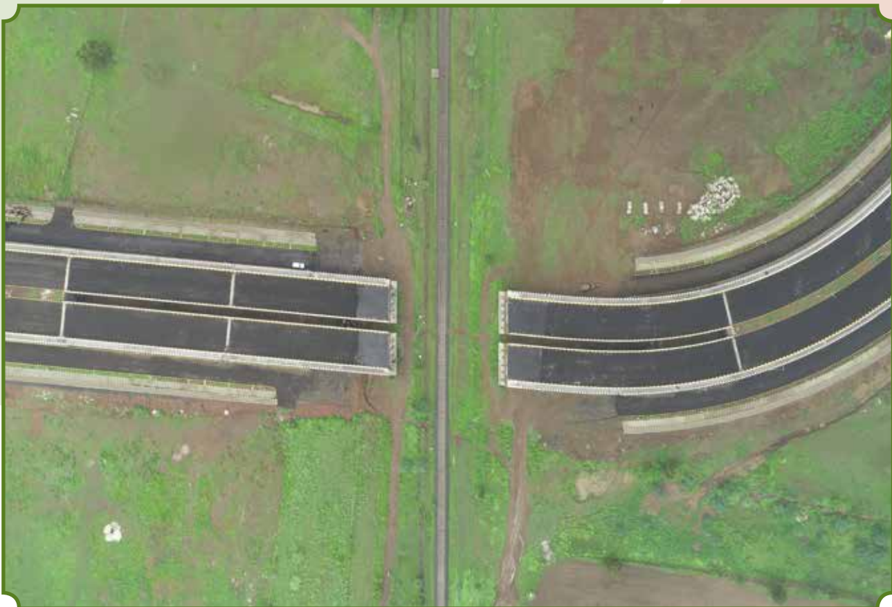
CONSTRUCTION OF RAIL-OVER-BRIDGES (ROB-1 & ROB-2) AT SHENDRA INDUSTRIAL PARK, MAHARASHTRA
