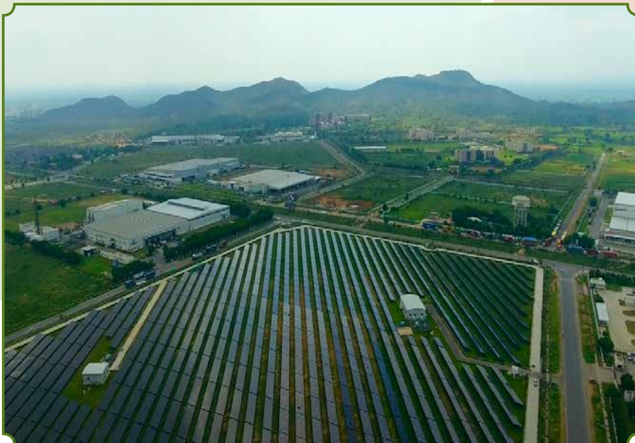
SOLAR POWER PROJECT AT NEEMRANA, RAJASTHAN
