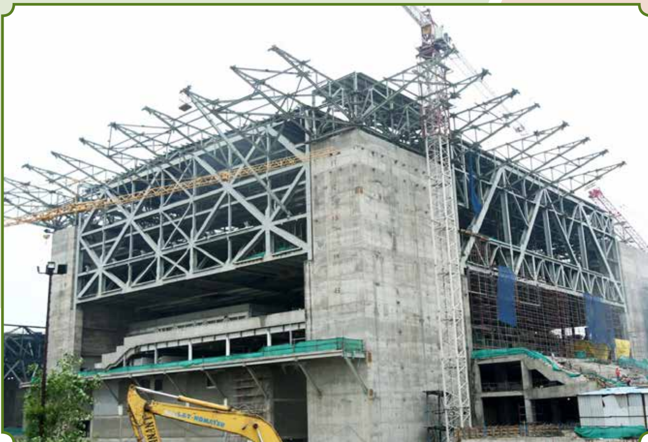
CONVENTION CENTRE – CANTILEVER ERECTION AT INDIA INTERNATIONAL EXHIBITION AND CONVENTION CENTRE AT DWARKA, NEW DELHI
