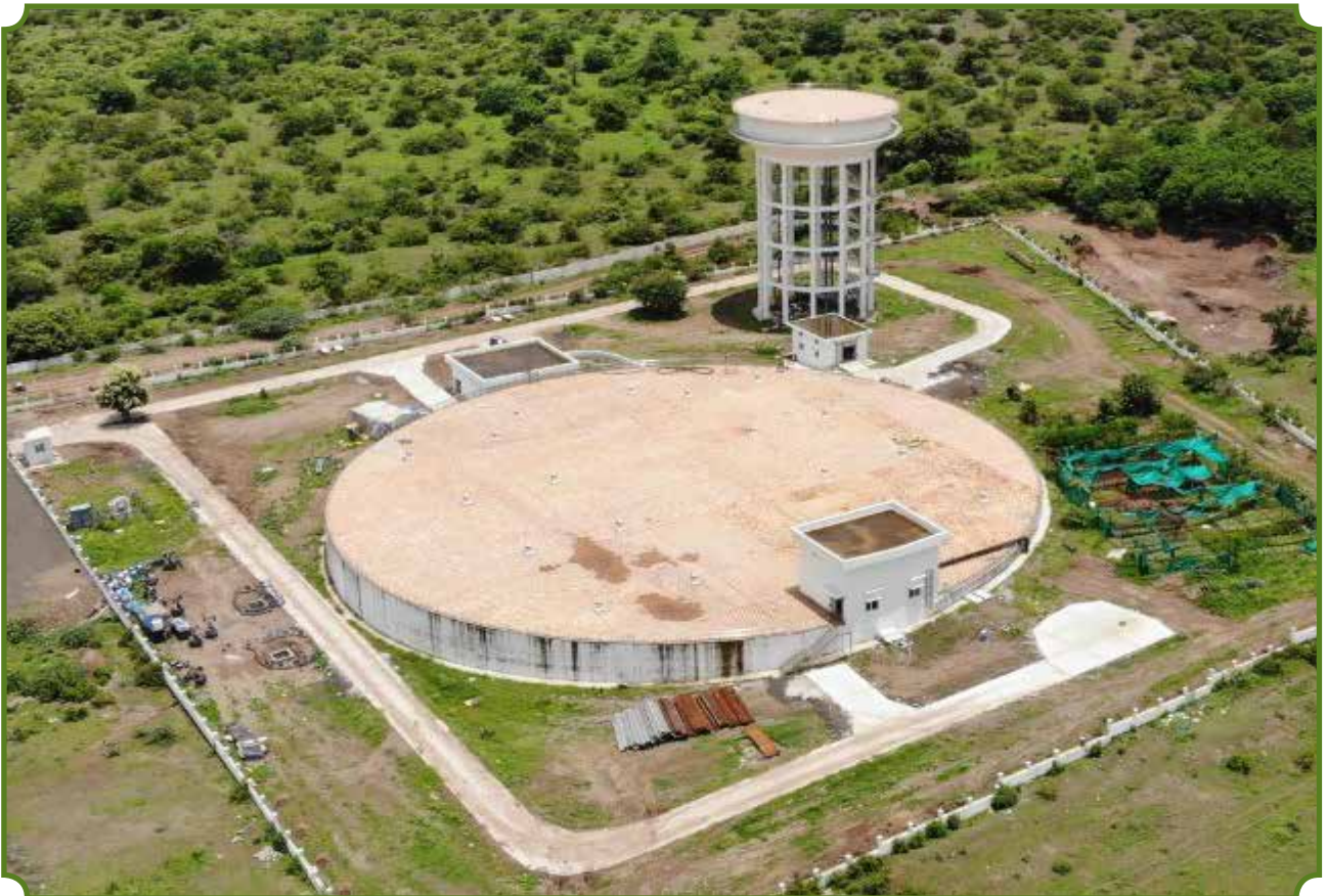
UNDERGROUND STORAGE RESERVOIR (UGSR) AT BIDKIN AND SHENDRA INDUSTRIAL PARK, MAHARASHTRA
