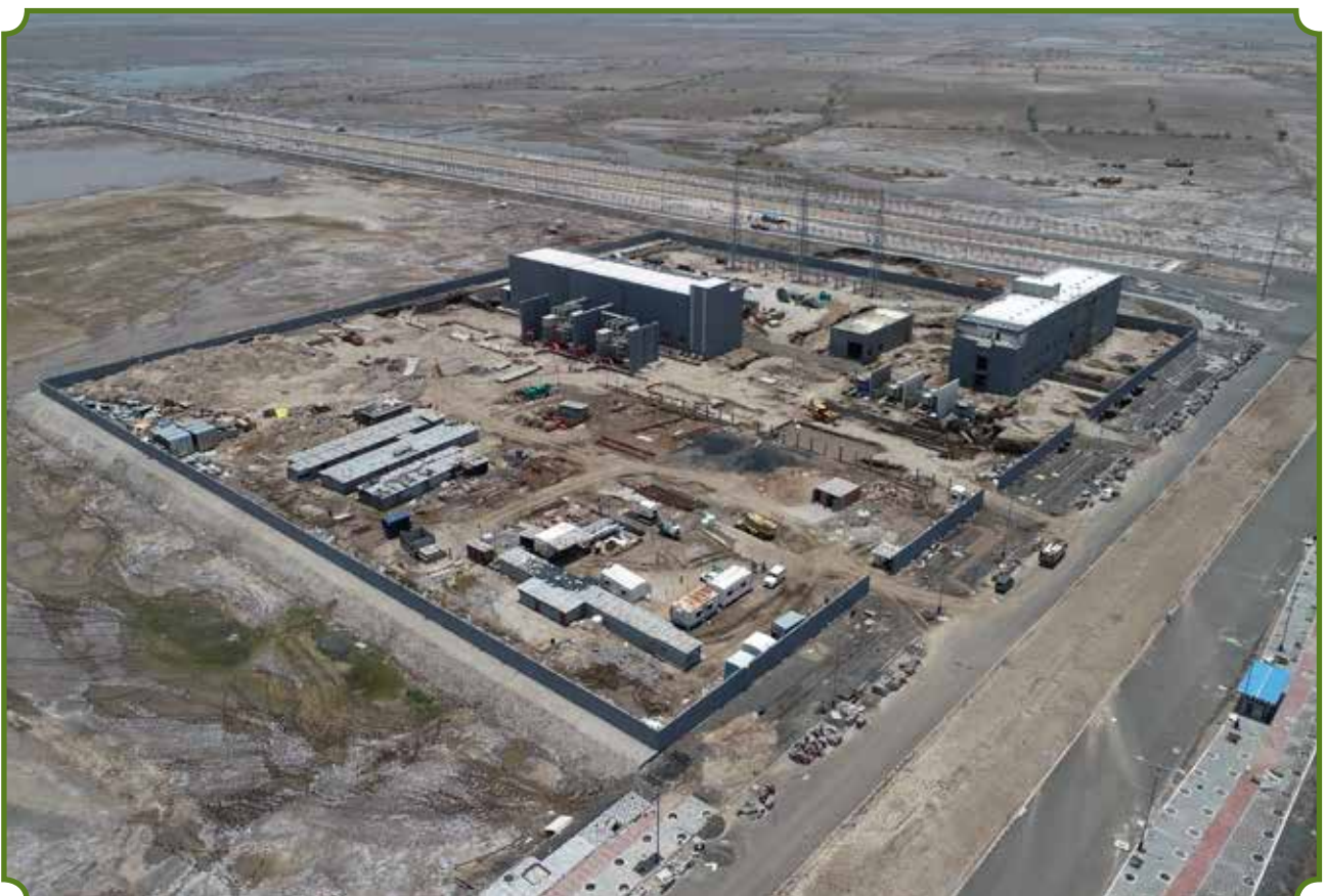
CONSTRUCTION OF COMMON EFFLUENT TREATMENT PLANT, SEWAGE TREATMENT PLANT AND POWER SUB-STATION AT DHOLERA, GUJARAT
