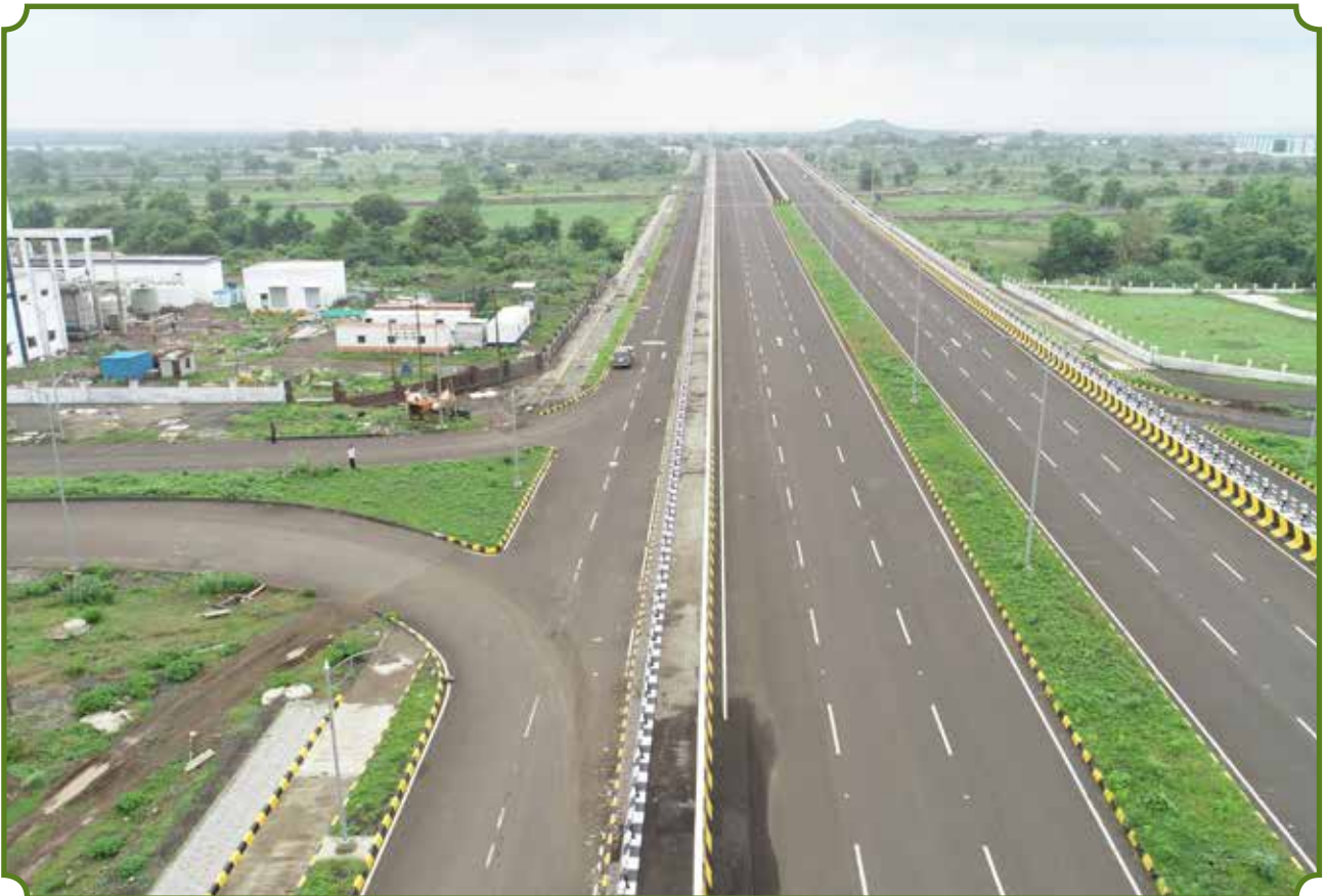
ROAD & SERVICES AT SHENDRA INDUSTRIAL PARK, MAHARASHTRA
