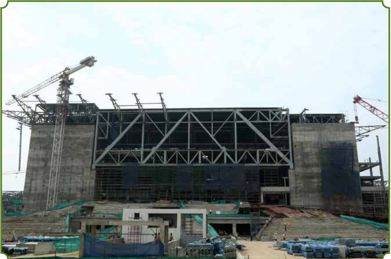
CONSTRUCTION OF CONVENTION CENTRE AT INDIA INTERNATIONAL EXHIBITION AND CONVENTION CENTRE AT DWARKA, NEW DELHI
