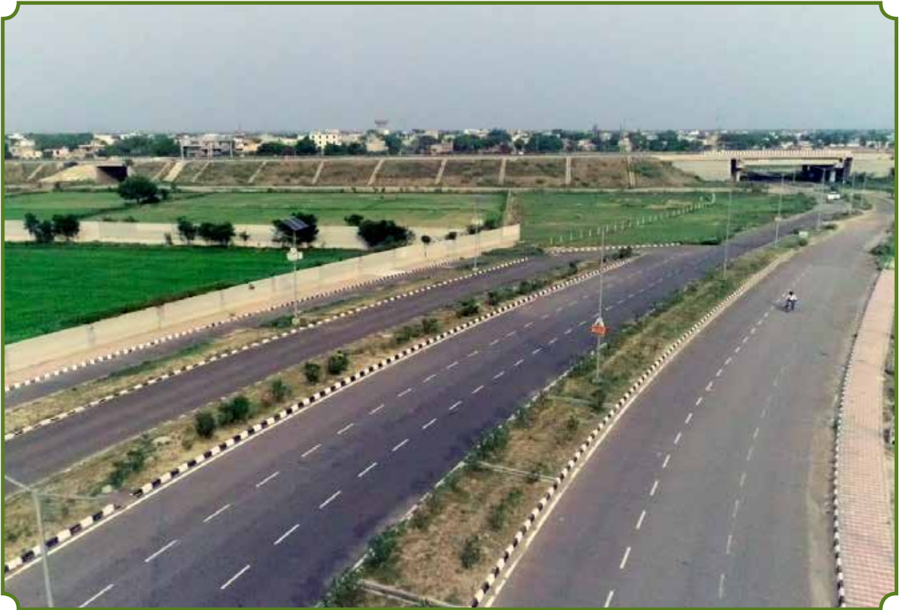
CONSTRUCTION OF ROAD AND SERVICES AT INEGRATED INDUSTRIAL TOWNSHIP AT GREATER NOIDA, U.P.
