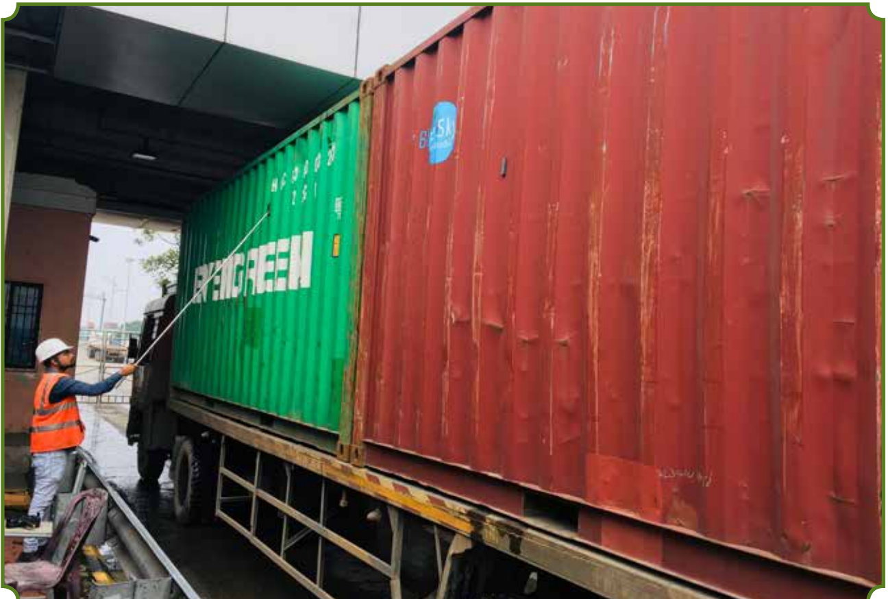
RFID READERS BEING INSTALLED AT TOLL PLAZA UNDER LOGISTICS DATA SERVICES PROJECT
